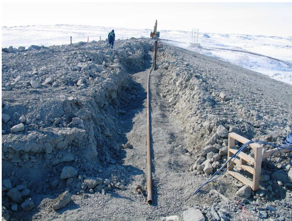
Photo 7: Positioning pipe in place .
