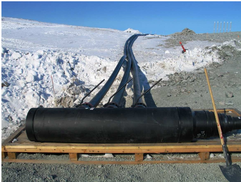
Photo 3: Termination of pipes on pad by Sta 0+60 thermister cable.
