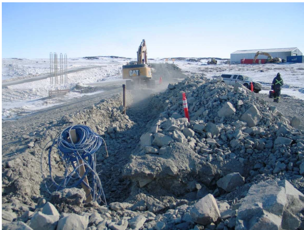
Photo 5: Excavation for connector cable, Sta 1+30 to Sta 1+75
