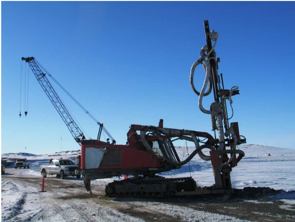
Photo 4: West Arc drilling thermister at jetty..
