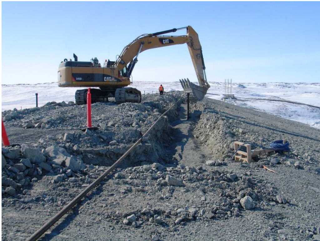
Photo 7: Positioning pipe in place .
